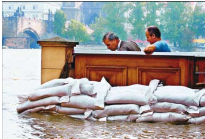
Finished dam barrier
