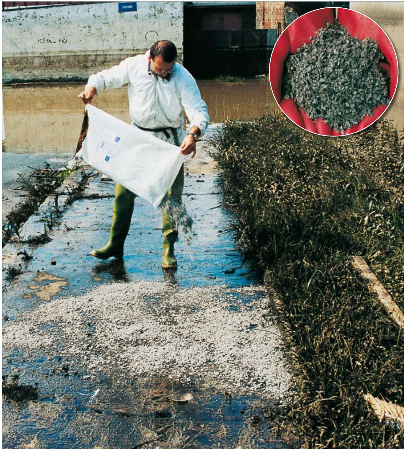
Removal of the oil leakage on ground
