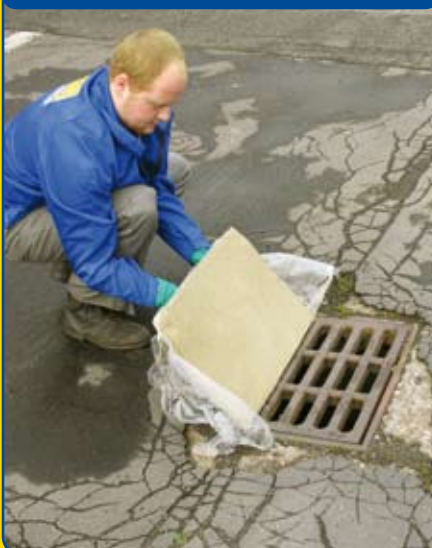
Spill tray without absorptive materials from ABS
