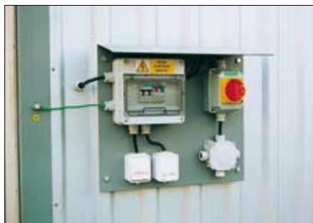
Lighting switch board
