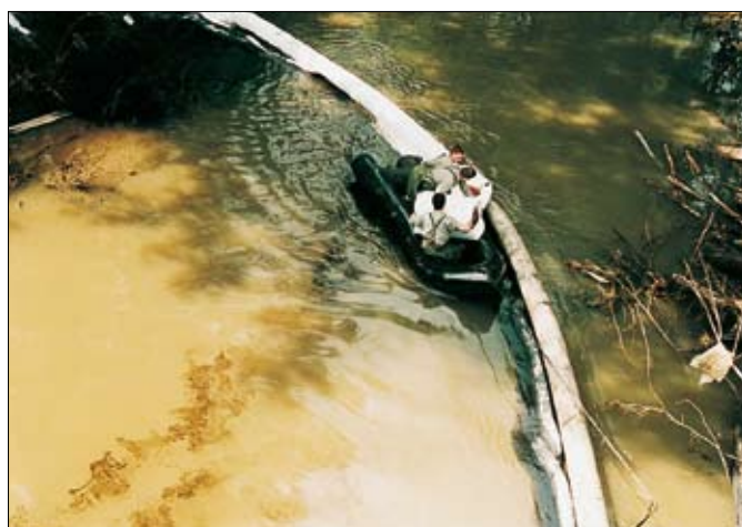
Efficiency increasing of a fixed spill containment boom by completing it with the absorptive mat
