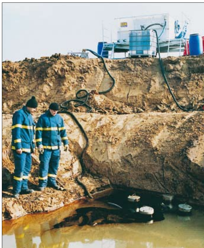
Mobile oil separator REO100 was used for a treatment of the oil phase from water surface inside the catch lagoons during the removal of the oil pipeline Družba breakdown in Čáslav on 9. 2. 2005.
